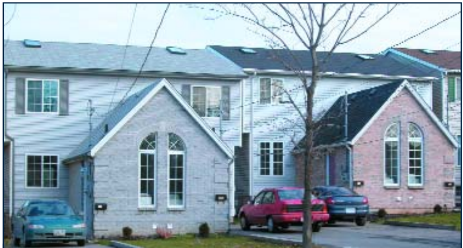
Dr. Tony Shaw of Brock University compared the thermal efficiency of two units in these nearly identical semi-detached homes. The house on the left was built with SIPs, while the other was framed with studs and batt insulation.
